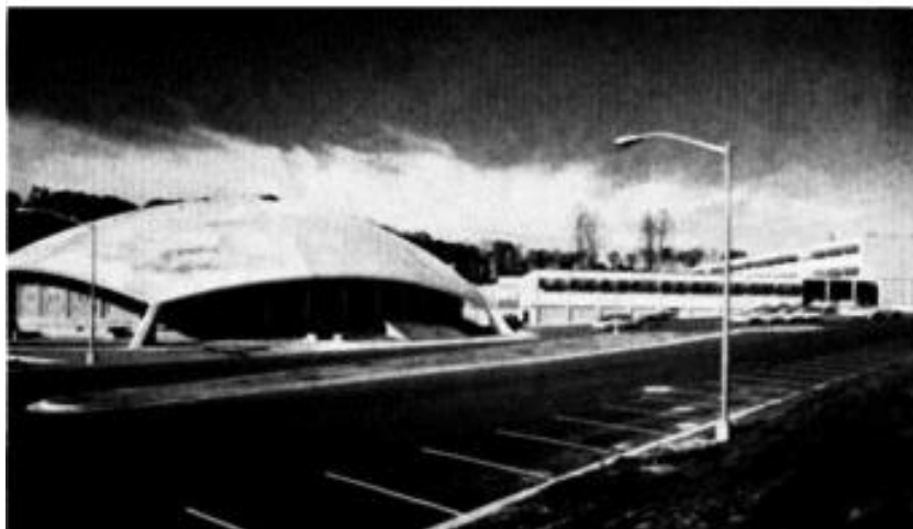
The geodesic dome is the principal design element in this new field house at Walt Whitman High School, Bethesda, Maryland (see story above).
